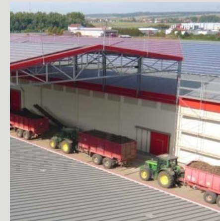
C&I system (greenfield): Oschersleben
