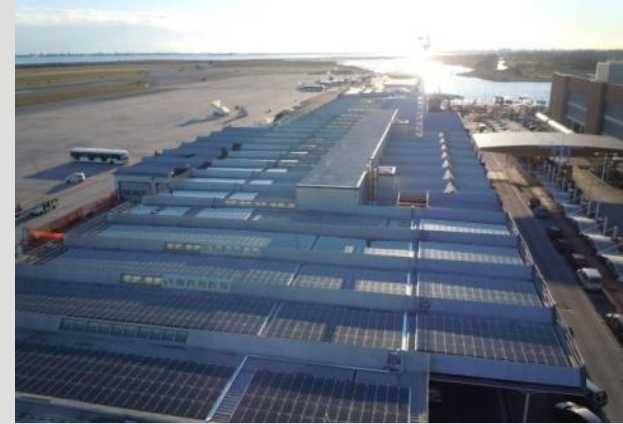
Rooftop installation Venice Airport, Italy
